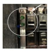
Line voltage wiring should be routed through the access holes at the top of the electric furnace. Proper electrical conduit connection fittings should be used. Connect the power wiring to the line side connections on the electric furnace. The electrical ground wire should be connected to the grounding lug. Ensure both the field supplied ground wire and electric furnace GREEN ground wire are both secured to the grounding lug of the electric furnace.
