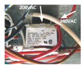
If the line voltage being supplied to the electric furnace is 208-volt single phase, the line voltage tap on the low voltage transformer needs to be moved from the 240-volt tap to the 208-volt tap. If this is not done, the secondary output voltage of the transformer will be too low.
